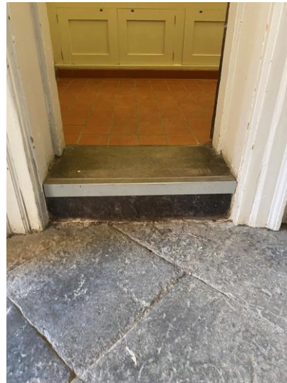
Step to enter men's toilets
