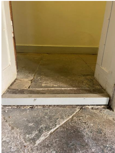
Step to enter women's toilets
